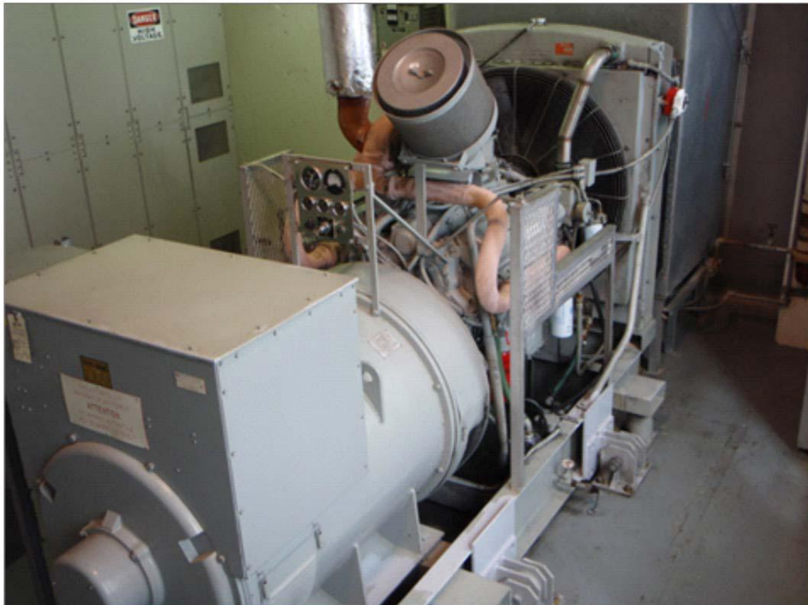
Figure 3-7. Diesel-electric generator set (source: Toronto International Airport)
