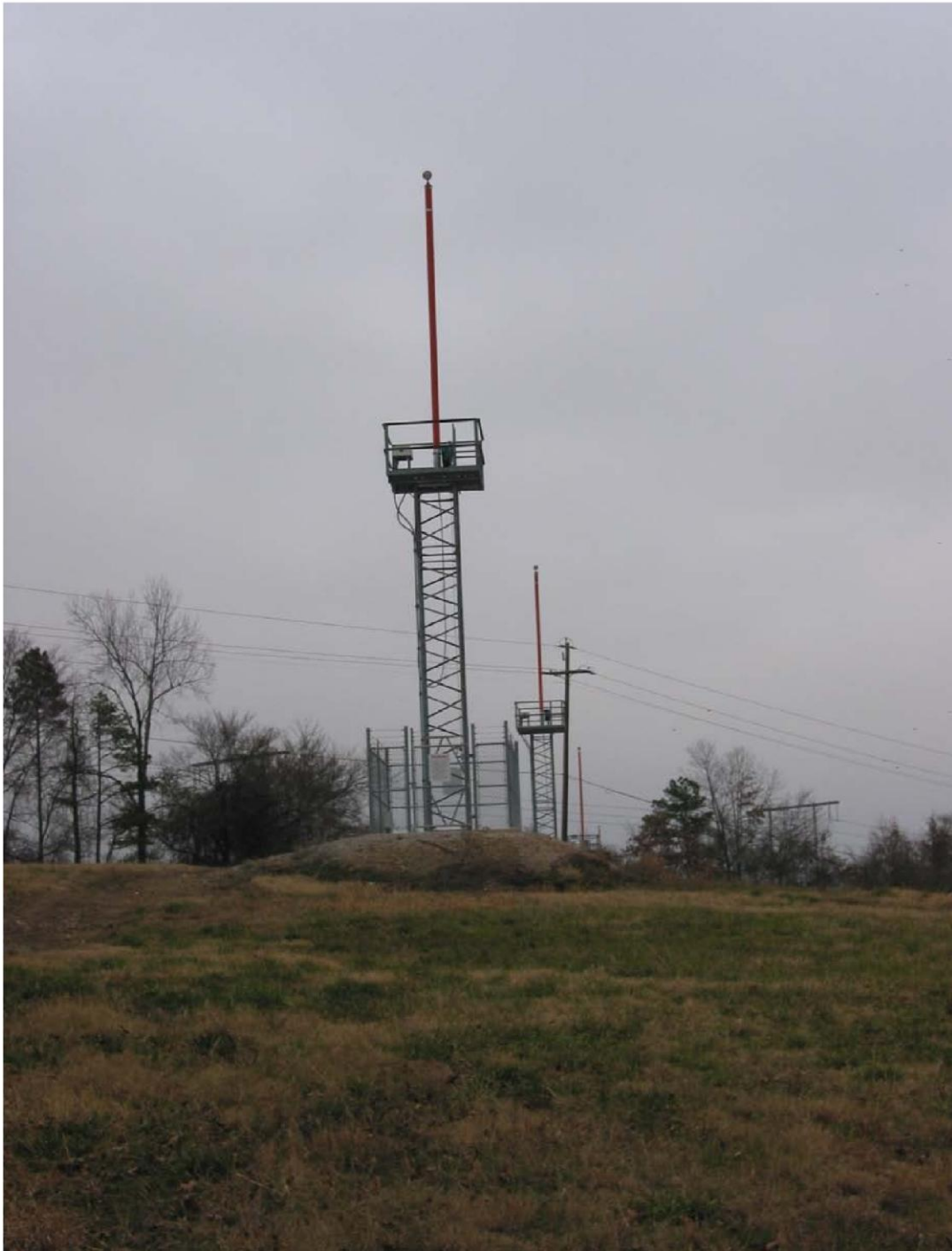
Figure 4-7. Fiberglass tubular pole on rigid structure
