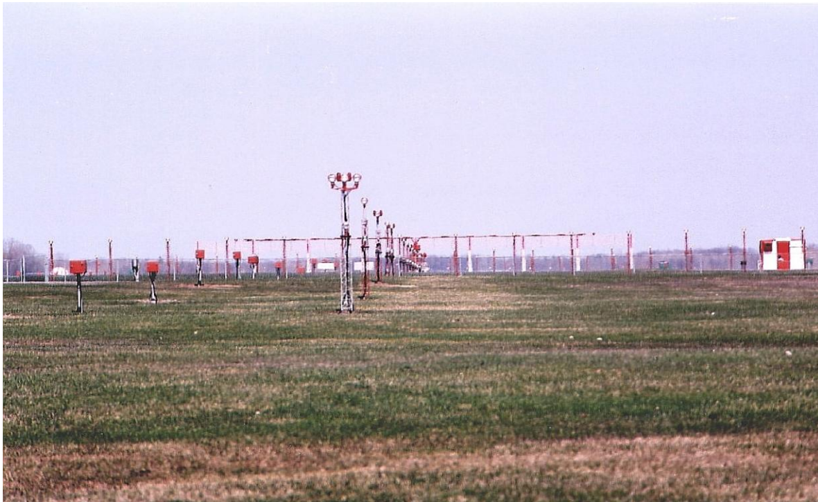
Figure 4-4. Approach lighting towers — aluminum lattice structures
