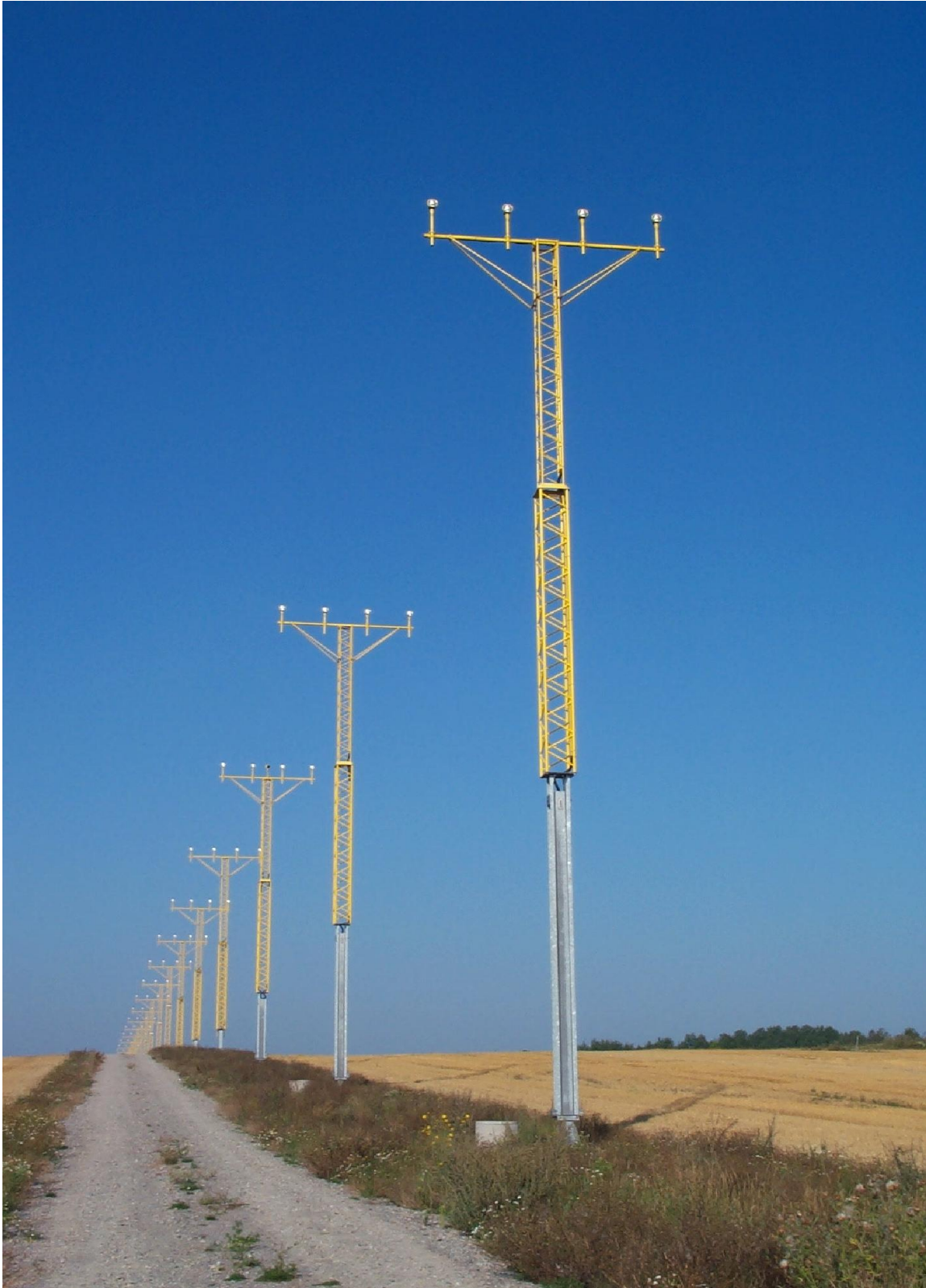
Figure 4-8. Fiberglass approach lighting towers on rigid supporting structures
