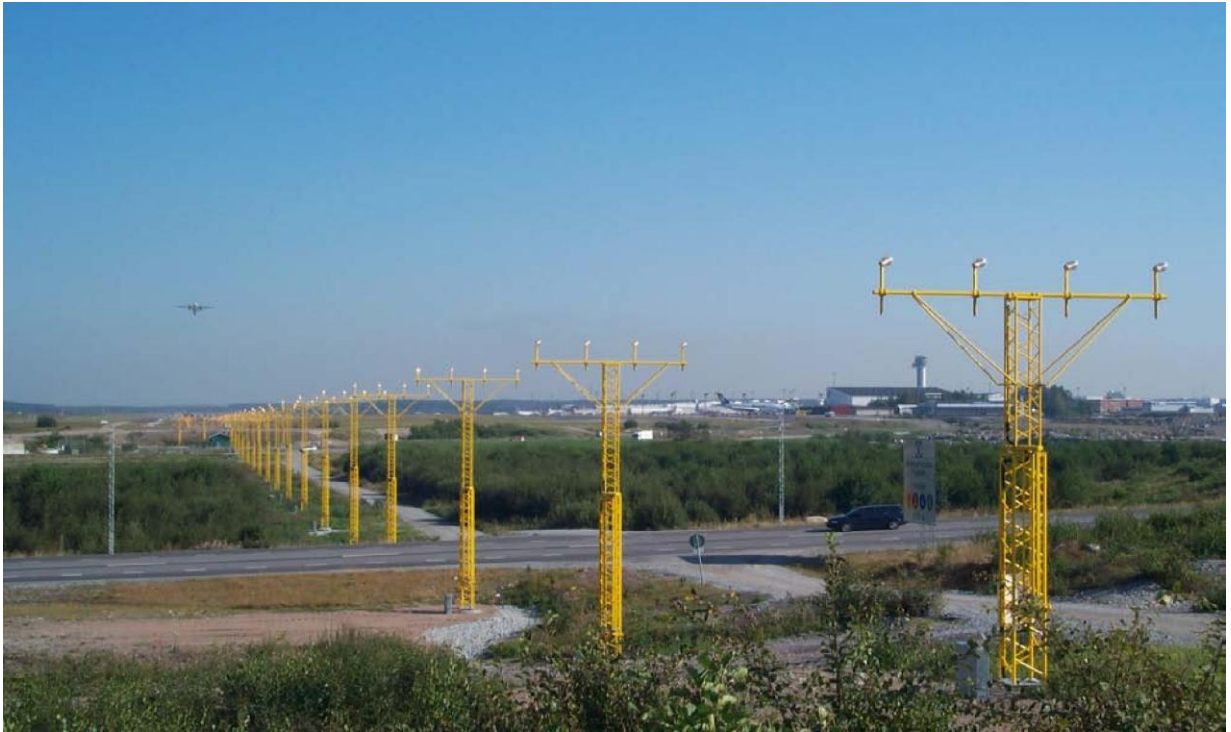
Figure 4-2. Approach lighting towers — fiberglass lattice structures
