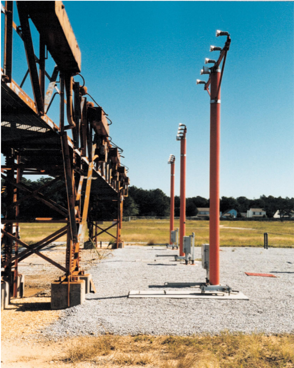
Figure 4-5. Close-up of an approach lighting tower — aluminum lattice structure
